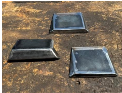
Surplus weld removed.
